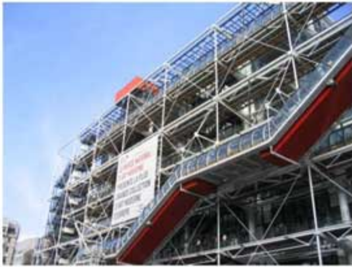
The Centre Georges Pompidou (constructed 1971 - 1977) Renzo Piano, Richard Rogers 1
