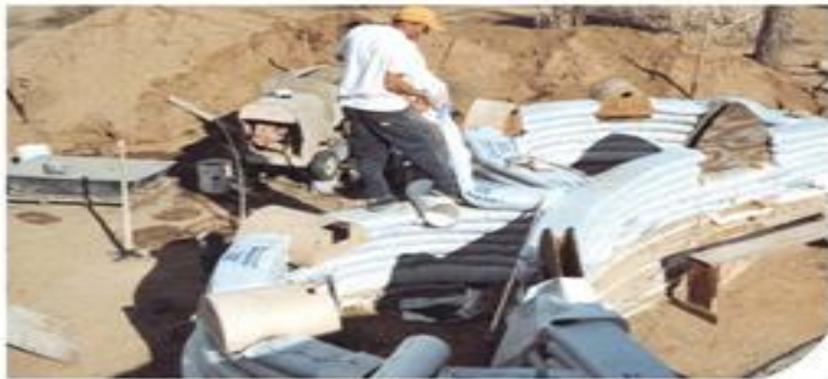
Demonstration of the construction of domes with multiple arches and rooms using the "superadobe" method that meets United Nations standards.
