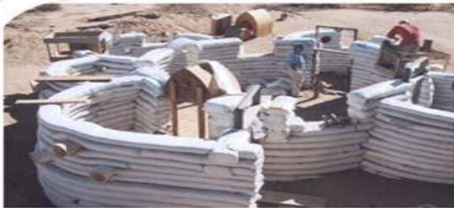
Demonstration of the construction of domes with multiple arches and rooms using the "superadobe" method that meets United Nations standards.
